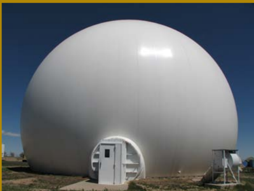
CSU-CHILL Radome and Airlock Entry
