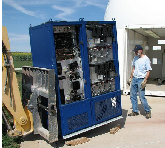
Figure 12: Raytheon ASR11 transmitter being moved to its operational housing, a customized 20 ft sea container.
